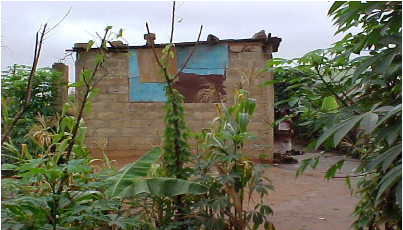
Figure 1 An Uncompleted House in East Legon
