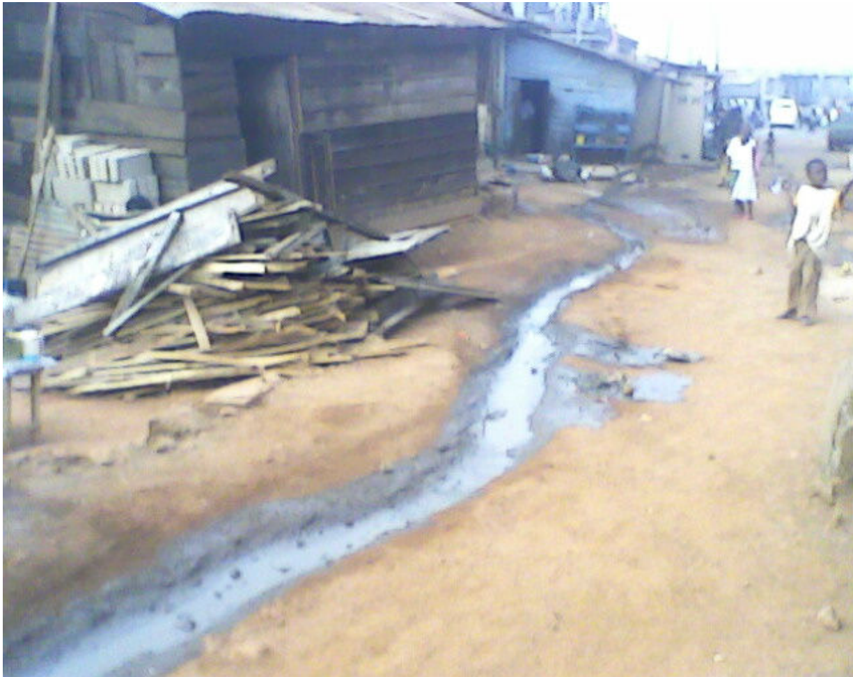
Plate 1: Evidence of unauthorised structures at Aboabo
